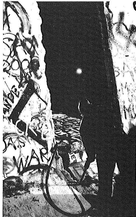
One of the most emotional symbols of the end of the cold war era was the demolition in November 1989 of the Berlin Wall, which had divided the city since 1961.
