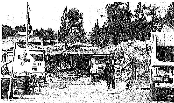
There was not much left of the U.S. Marine headquarters in Beirut following the terrorist bombing in 1983.
