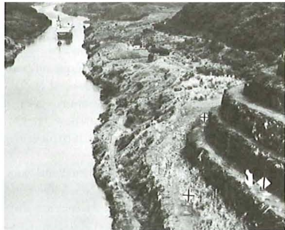
Daybeacon ranges in the Gaillard (Culebra) Cut of the Panama Canal. Pilots conning ships transiting the canal do much of their steering through the canal on these daybeacon ranges.
