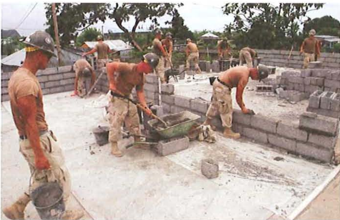
Seabee personnel construct a six-room schoolhouse in Maroni, Camoros, in support of the humanitarian assistance element of U.S. maritime strategy as set forth by the chiefs of the maritime services in 2007. (Kenneth Fidler)
